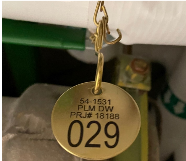
Figure 2: Valve tag installation.
